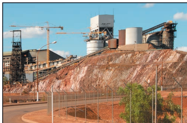
Figure 13. Mine buildings above an old open pit at Mount Isa.
